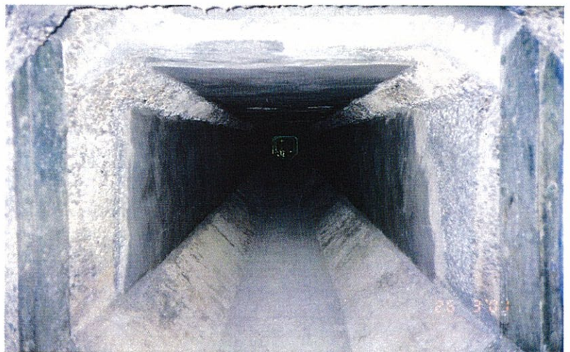
Application of 3 pack epoxy mortar to all internal surfaces with areas sectioned off.
